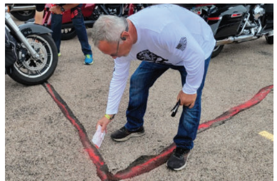
"Vegas" filling in the cracks
